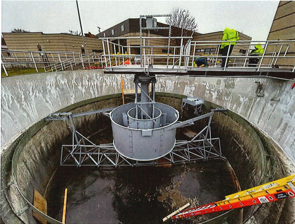
Figure 3: New Clarifier #1 equipment installed
