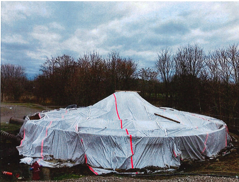
Figure 2: Painting of digester cover
