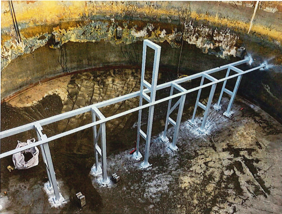
Figure 1: Cleaned and painted existing supports that were re-used in the digester
